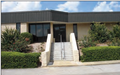
Olive Branch, Mississippi, USA Manufacturing and Distribution
