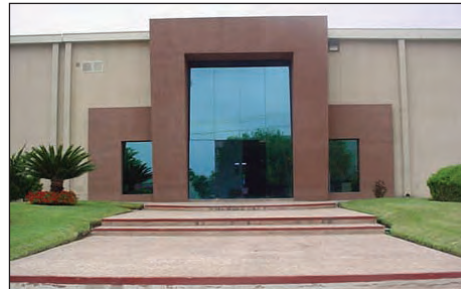
Monterrey, Mexico Manufacturing and Distribution
